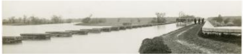
RICHMOND AQUEDUCT - PHOTO ENHANCEMENT BY BILL HECHT
